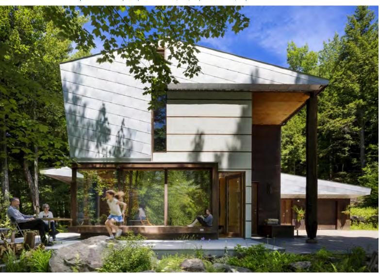
materials; there are no painted or stained walls inside and no carpeting because of the radiant-heated floors. Dunbar suggested low-maintenance building materials—plywood, concrete, tin, Vermont slate and knotty pine—that evoked local landmarks, such as woodsheds, barns and mountain lodges.
